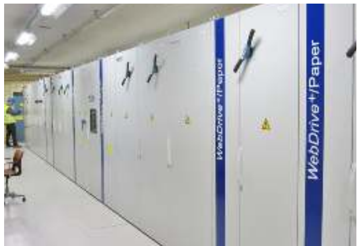
Fig. 8: Switch cabinets for WebDrive+/Paper
